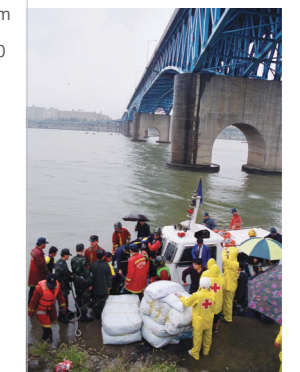
1994 Emergency relief at Seongsu Bridge collapse site
