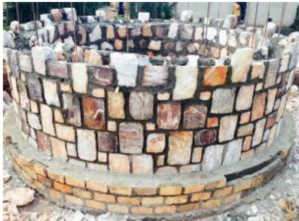
Foundation for two kiosks are constructed
