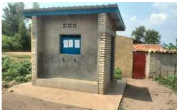
The constructed water Kiosk
