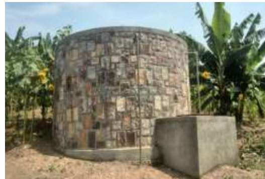
The constructed water storage tank
