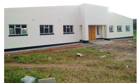
Completed Evacuation Centre at Manzvire, Chipinge District
